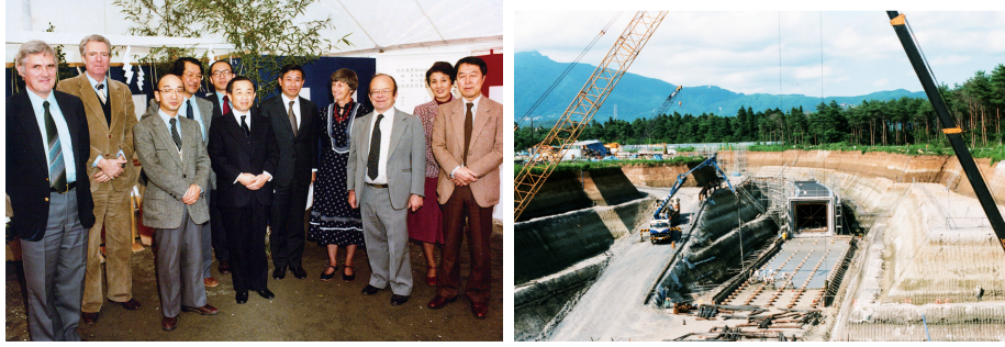
Figure 1: (left) Groundbreaking Ceremony of TRISTAN on Nov. 1981, attended by S. Ozaki, T. Nishikawa, Y. Yamaguchi, P. Panofsky, Y. Nambu. (right) Accelerator tunnels and experiment halls were constructed open-cut. Mt. Tsukuba at the back.
