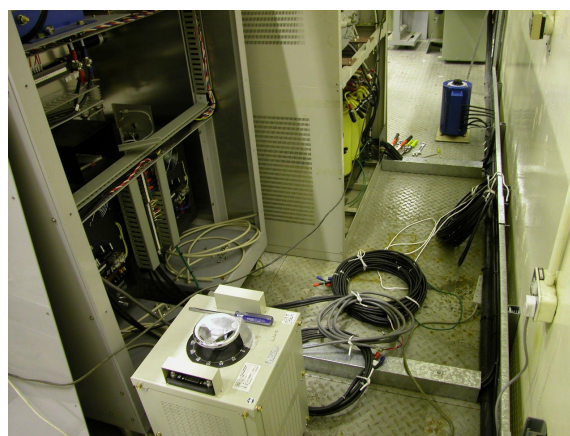
Photo 2: Wired output cables.
