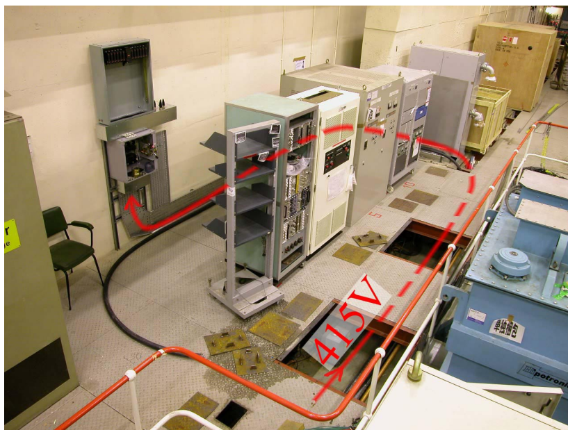
Photo 1: Preparation for AC power distribution
