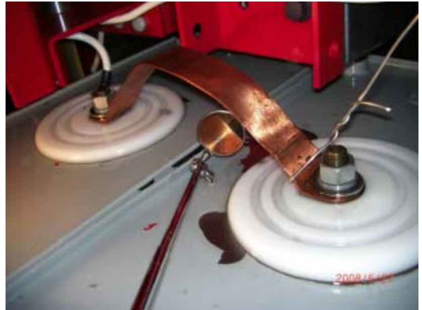
Flashover of the output capacitor
