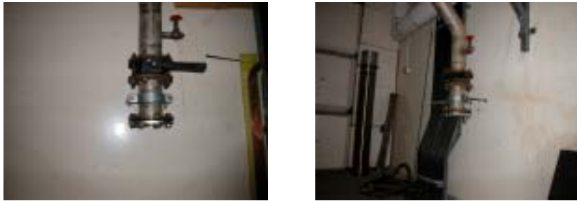
Figure 3. Water connections in the MICE Hall in the opposite side of the trench.
