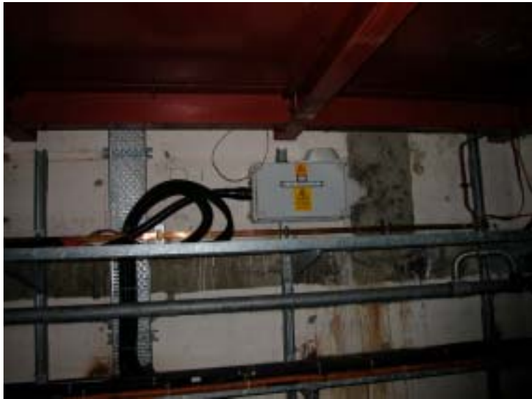
Figure 2. Present power-distribution-unit along the wall at the trench side.
