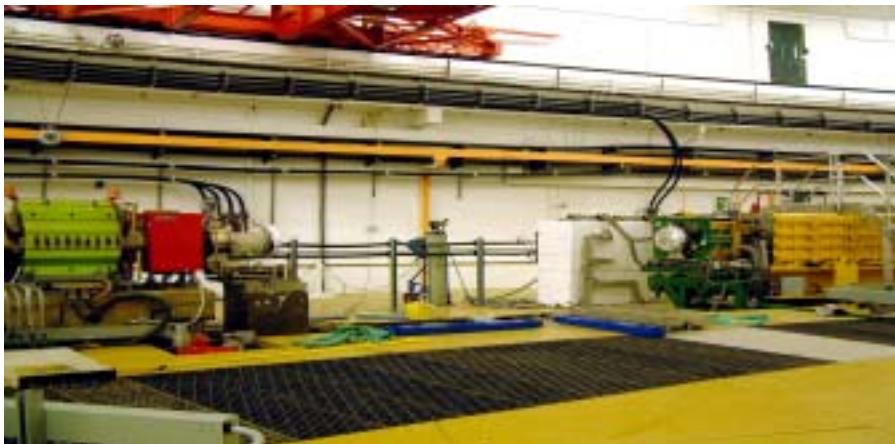
SP6 with components removed and new base supports being installed
