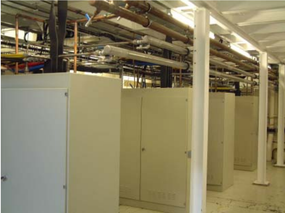
View of the four Bias Transistor Regulators
