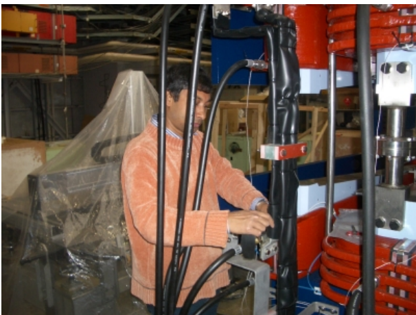
Figure 7: Busbar 絶縁作業
