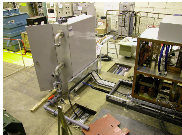
Photo 7: Cables from LOI Control Console through a pit
