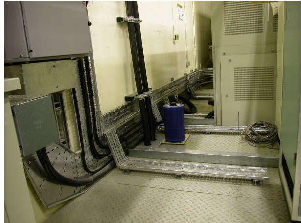
Photo 6: Power Lines to Power Supplies
