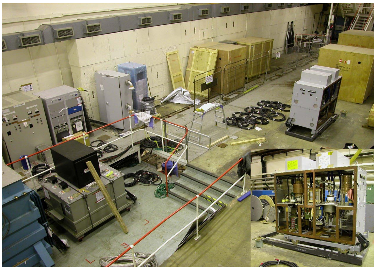
Photo 1: MICE Hall and HPD on a rail.
