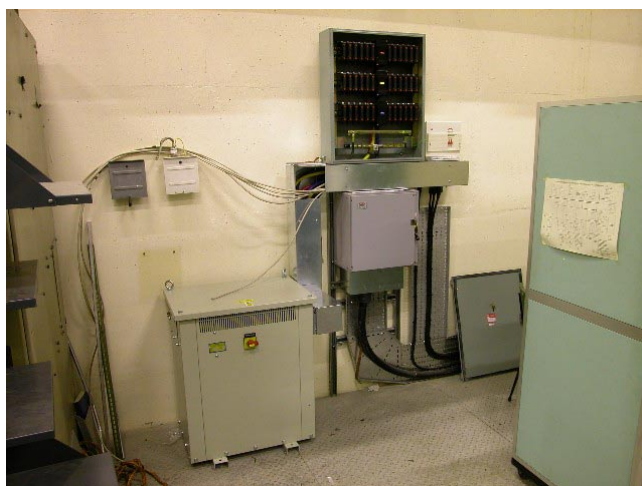
Photo 2: 60 kVA transformer
