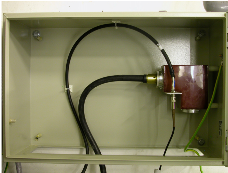
Figure 3. Breakout box 2 for the tetrode anode and screen supplies.
