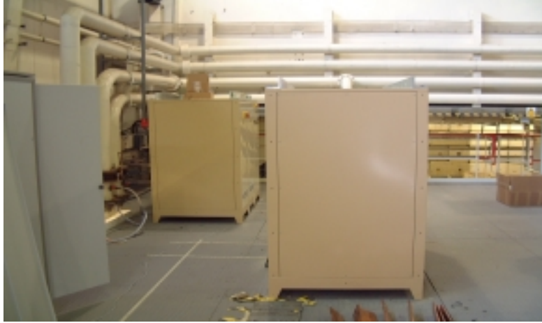
Hall 2 platform with two of the LVPS for the Bias systems.
