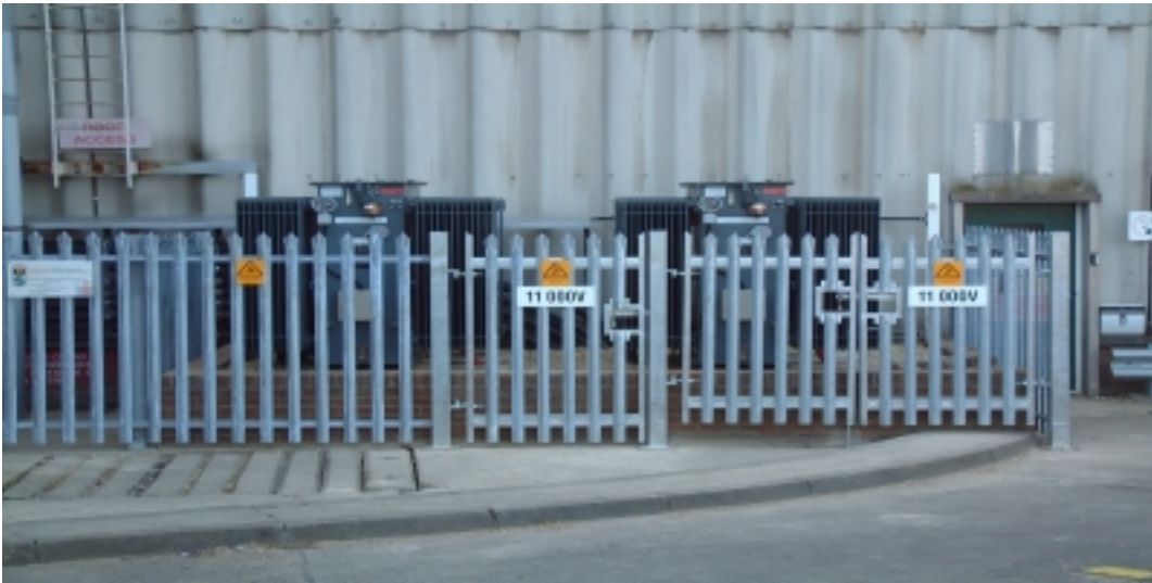
The new outdoor transformer bay showing two of the four 1.5MVA transformers
