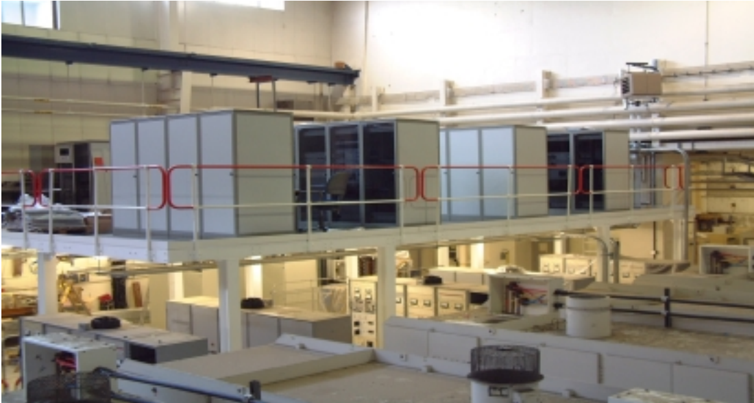
Hall 2 platform with racks for the HPD power supplies and controls
