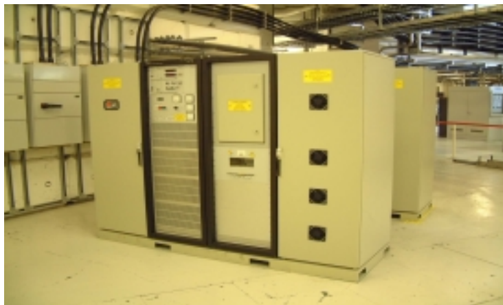
Two of the high voltage anode power supplies in Hall 2.
