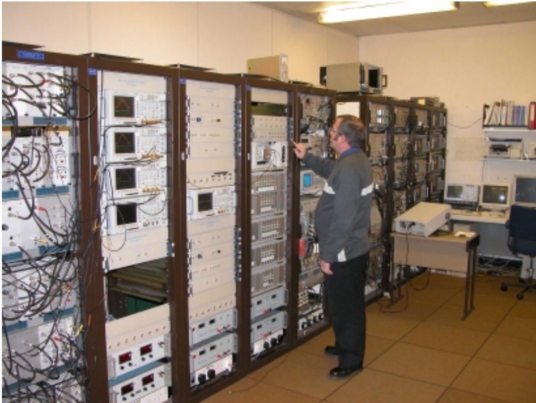
The LPRF rack layout adjacent to the main control room
