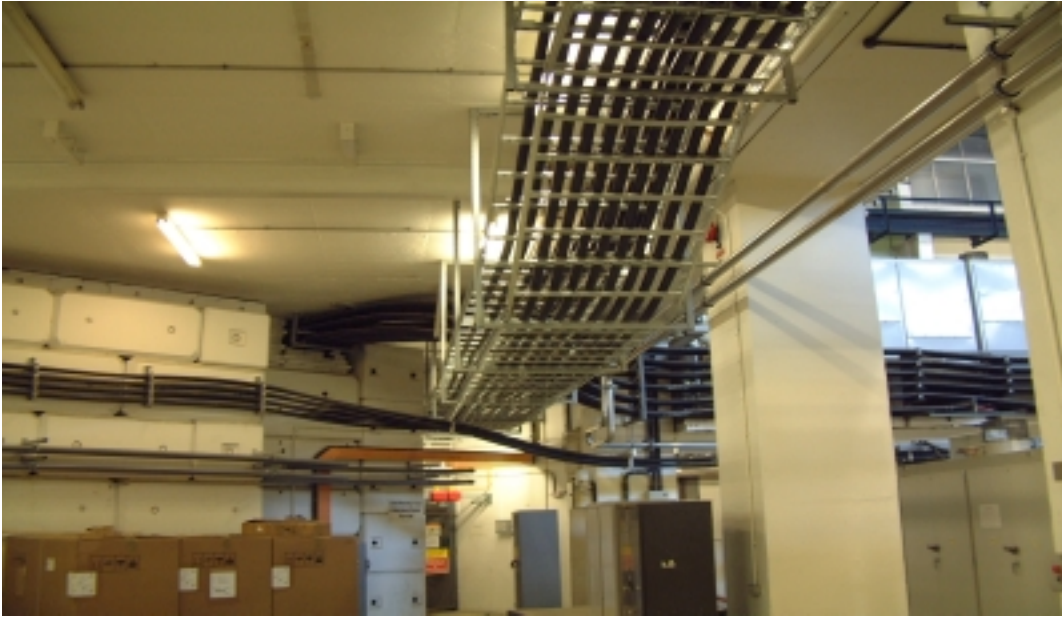
The sixteen, 4-core aluminium cables that run from the Bias Systems to the cavities.
