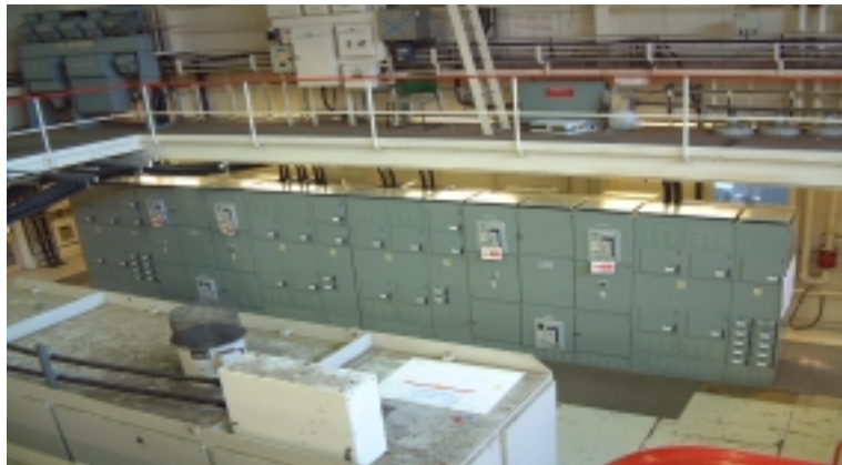
New 415V distribution board in Hall 2 (R5.4)
