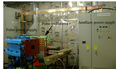
Figure 4: Auxiliary power supply has been connected to the pulse power supply in parallel at the primary winding of the matching transformer.
